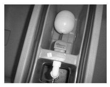
**Step 8**Connect your float assembly to the valve and adjust your water level to the desired height.
